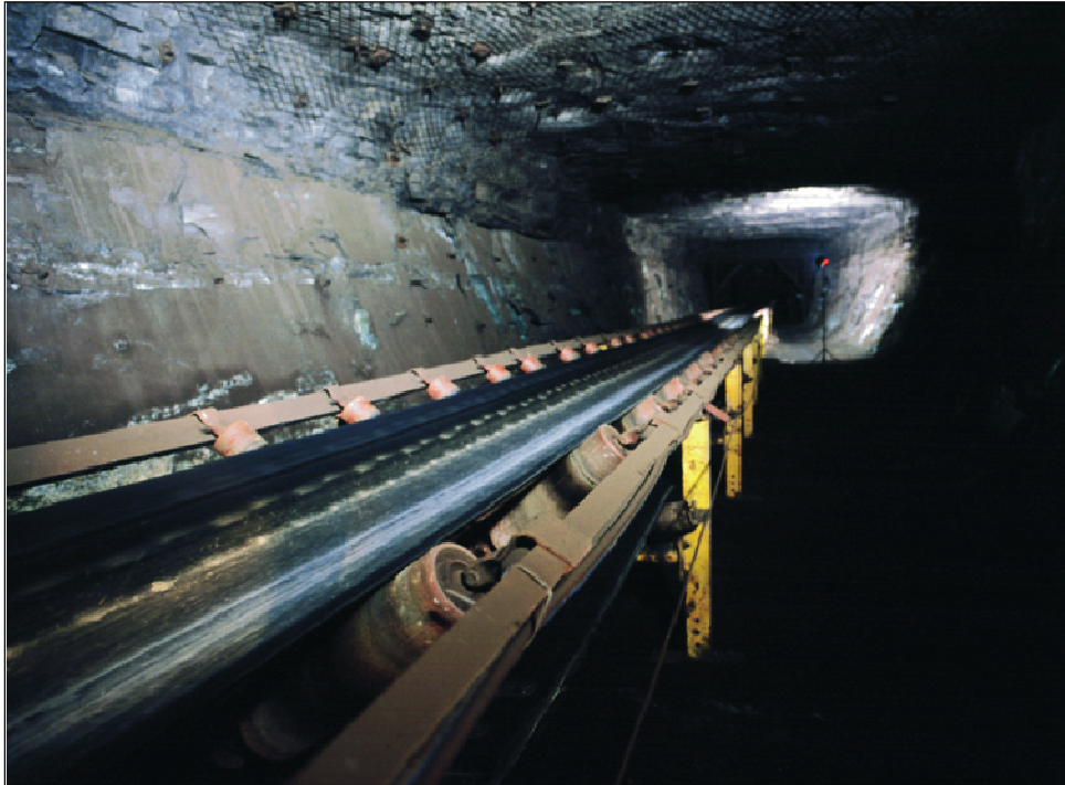
Figure 16.15 Typical Underground Conveyor
